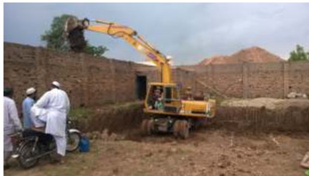
KK new office under construction.
